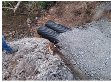
REPAIR OF COLLAPSED CULVERT AT HOLLYMOUNT, PETERSWELL
