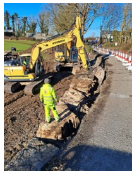
BEFORE, DURING AND AFTER PHOTOGRAPHS OF ROAD REPAIRS ON THE L-4509 FOLLOWING THE FAILURE OF A RETAINING WALL STRUCTURE
