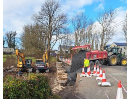
BEFORE, DURING AND AFTER PHOTOGRAPHS OF ROAD REPAIRS ON THE L-4509 FOLLOWING THE FAILURE OF A RETAINING WALL STRUCTURE
